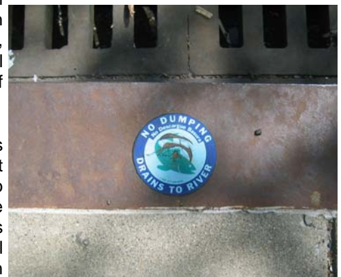
Existing Catch Basin Stencil
